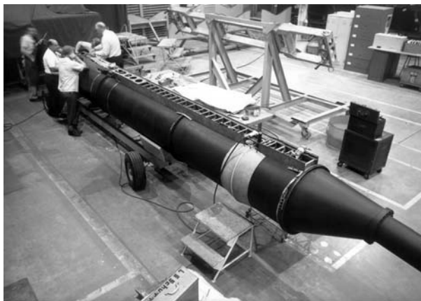
Figure 6. Initial application of aerodynamic ring.
