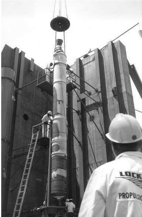
Figure 16. Technicians secure the booster (note the melting frost on the case exterior).
