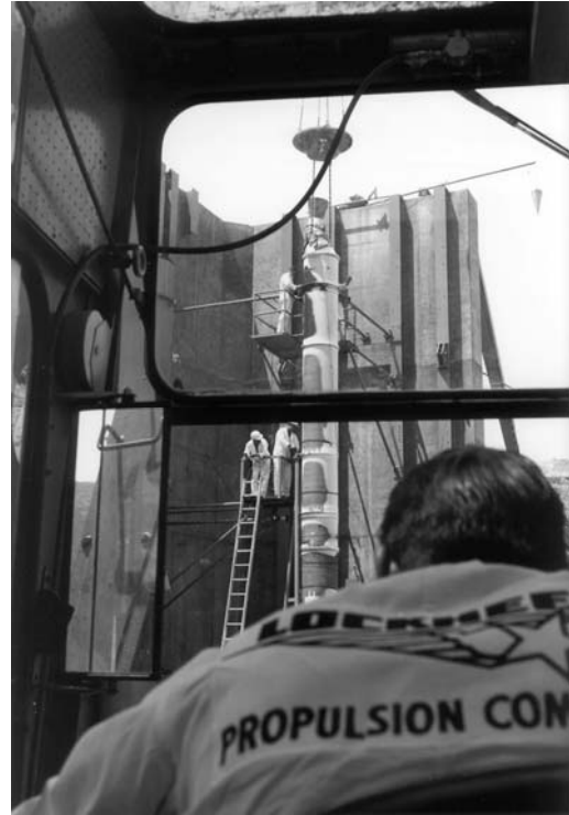
Figure 17. Crane operator's view.
